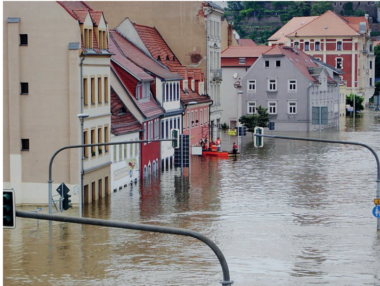
Fig. 17.2: Flood in the Urban Area.
